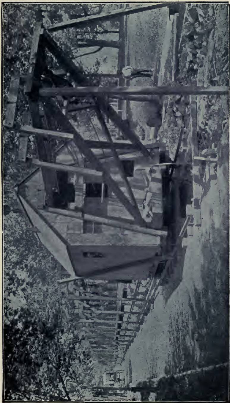
PLATE XII.—TRESTLE EXCAVATING-MACHINE AT WORK.
